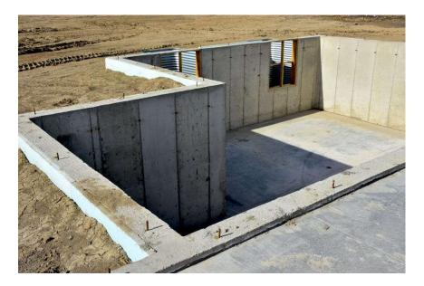
Though the basement adds additional space to the house they are types of house foundations that increase the cost of construction. Further, there are possibilities of occurring cracks in basement walls.
