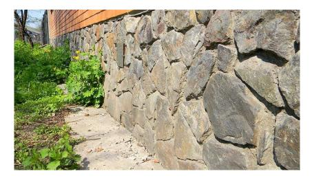
There is some sort of mortar in between the stoned to maintain the bond between the stone and mortar. Those structures are more durable and stronger.
